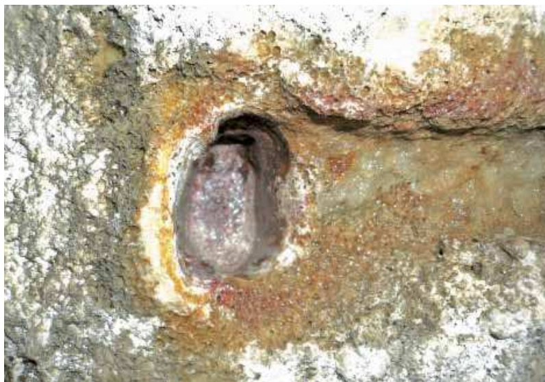
Fig. 3. The bed of vertical Π-shaped metal clamp preserved on the back of the torso of the statue of Hermes. NAM 2774.
